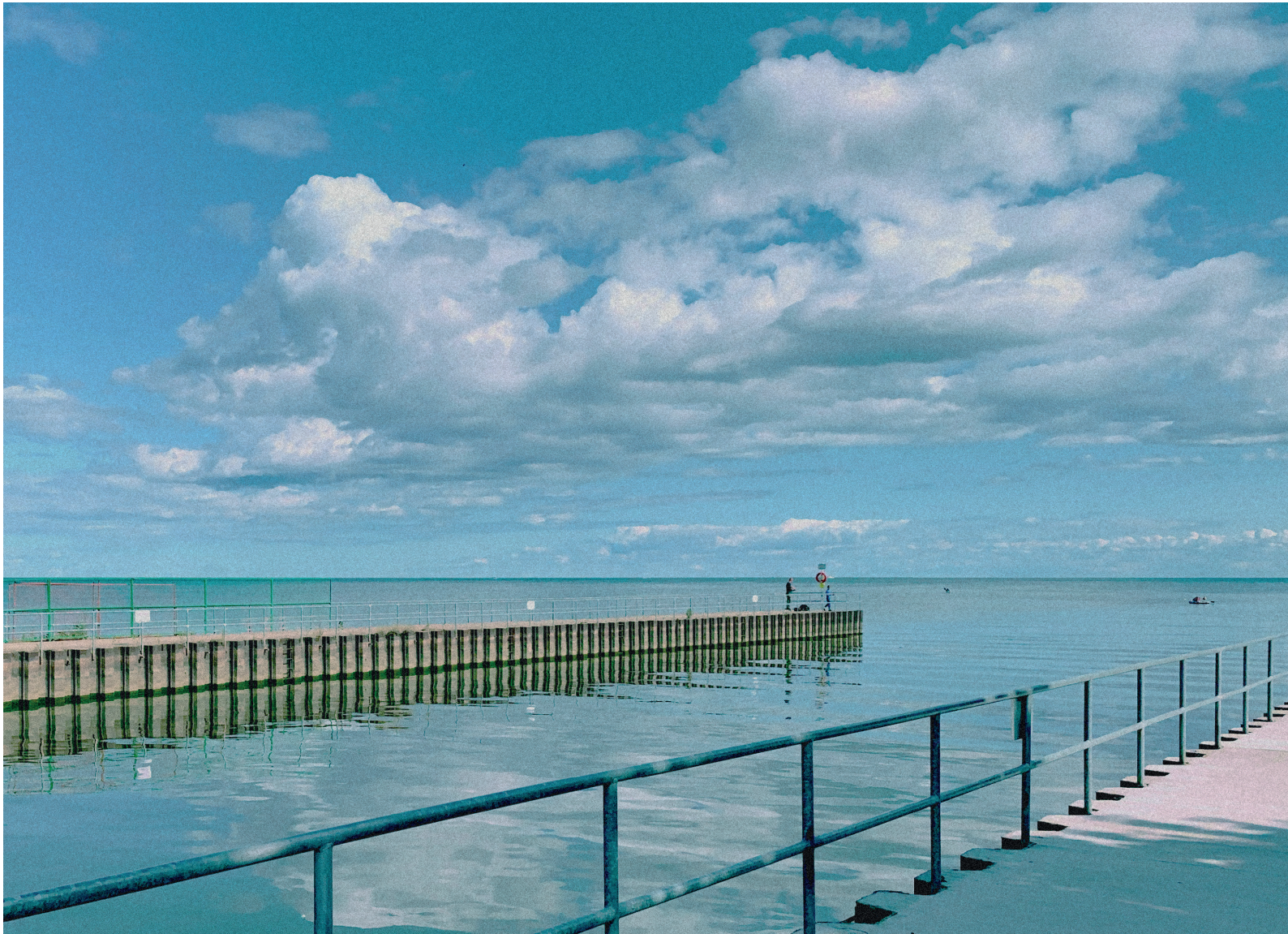
Pier | Photograph | September 2021
